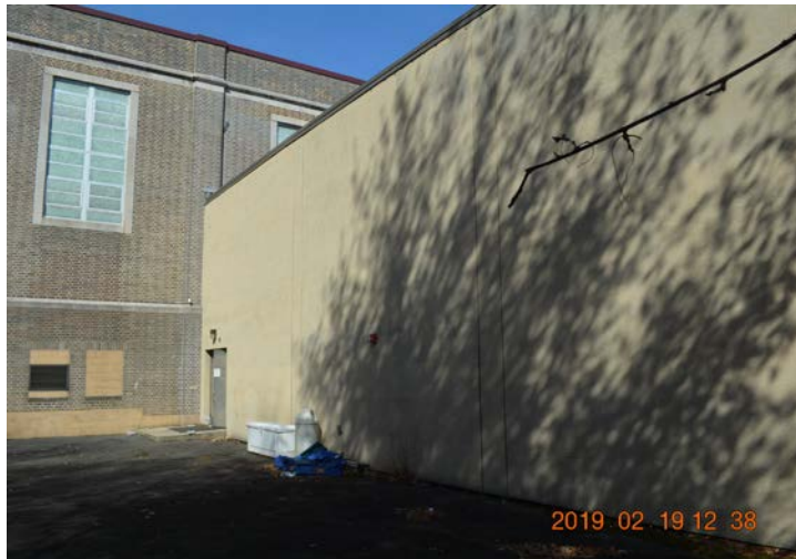
Photo 1: The 1980 Pool Addition was built up against the south wall of the 230 Gym that had been built in 1922. This is the wall facing Elliott Place. The pool exit doors are at the far edge.
