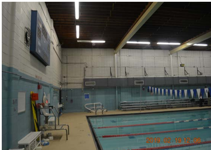
Photo 2: Just inside the double doors in the photo above, the 239 Gym exterior wall has been painted. The columns supporting the main girders above are located up against the original building's exterior wall.
