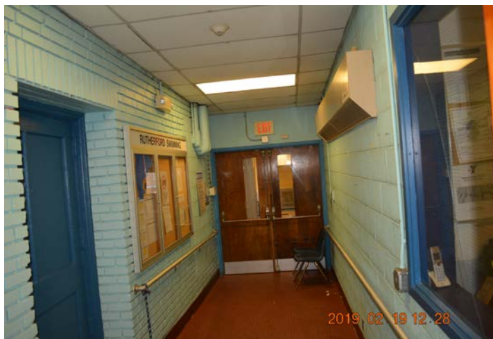
Photo 21: Existing corridor out to Locker Rooms and Showers, located through the end doors and to the left down a second ramp. Rubber flooring with raised disc tread pattern is moderately worn.
