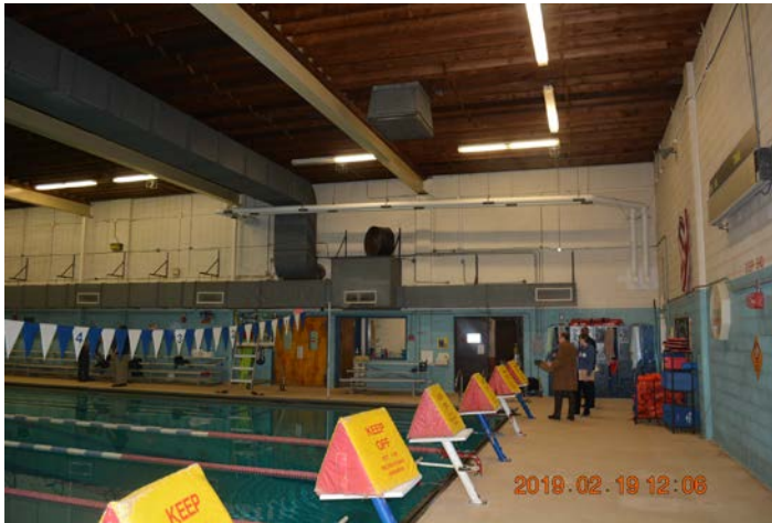
Photo 4: Pool Enclosure Interior Windows & Doors
