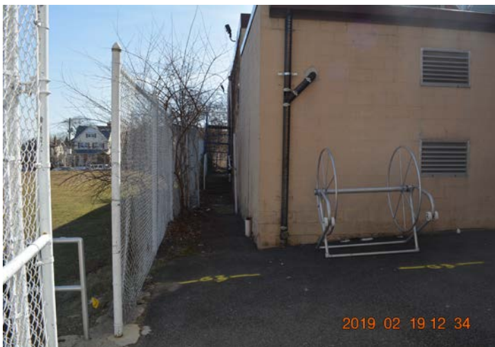
Photo 6: Backing up from the previous view, the wall of the Boiler Room and Filter Room beyond are exposed concrete masonry (CMU) walls, painted. They do not have the EIFS applied finish like the pool enclosing walls have.
