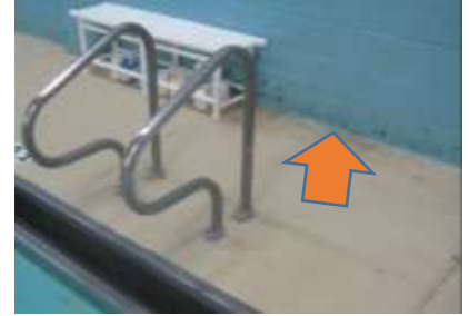
Deteriorated Paint
