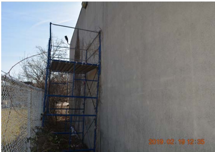
Photo 5: The east wall faces the field with distance to the fence line restricting access at this side also.
