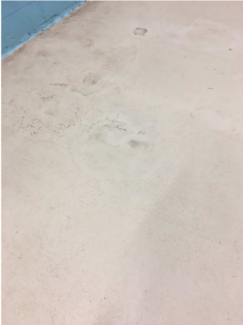
Photo 3 – Repair in pool deck with start of spall.
