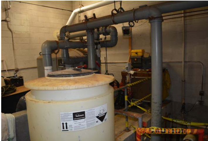
Photo 14: Filter Room, view of filter and water quality equipment arrangement.
