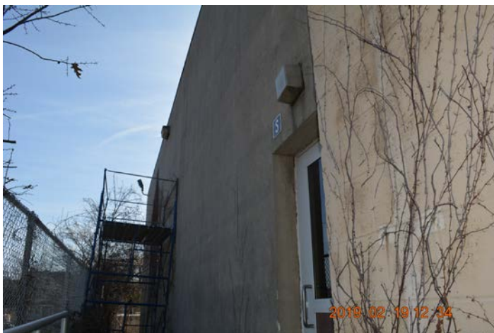
Photo 3: Pool facility exterior EIFS & CMU block wall transition. The pool enclosing walls have some insulating value from the EIFS. The exposed CMU walls around the support spaces seen in the right side of this view have little thermal resistance, and are not compliant with current Energy Conservation Code requirements.
