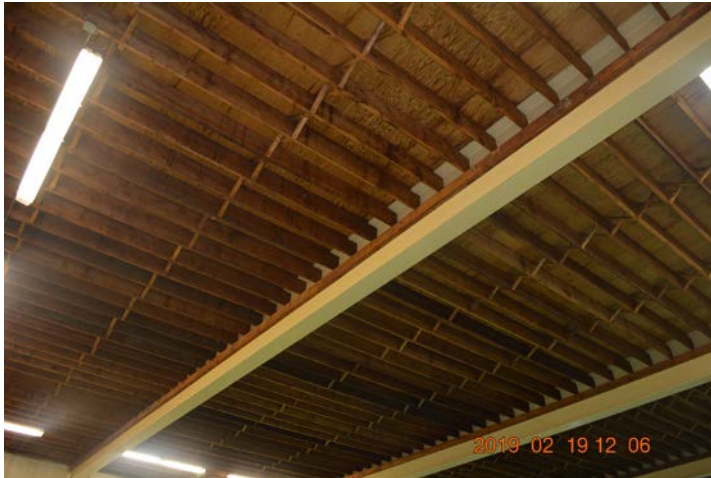
Photo 1: Pool roof structure is wood framed with plywood decking, exposed to view over the pool space.
