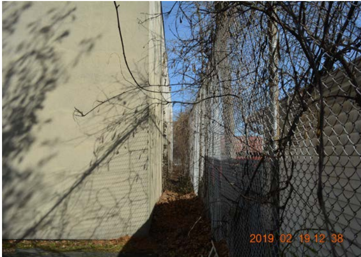
Photo 4: The south wall is very close to the fence at the property line, providing only limited narrow access to the surface for maintenance or renovation work.
