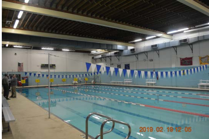
Photo 10: Main Pool Space Interior View: Main girders cross the space. Wood roof rafters span to ledger blocks on the beam sides. The pool has six lanes, with the starter platforms visible at the far pool end. Three tiers of metal bleachers are just off the photo to the left side. Existing supply ductwork is wall mounted at both side walls. General lighting is located only along the edges, where the fixtures can be serviced from the side deck areas.
