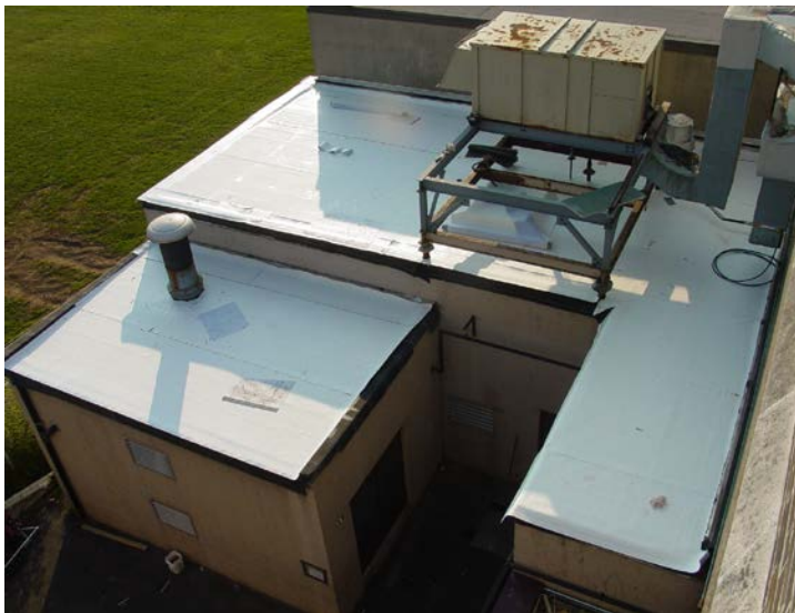
Photo 8: View of the new roofs over support spaces as they neared completion with the white reflective membrane. The replacement occurred only over the support spaces, and not over the main pool roof.
