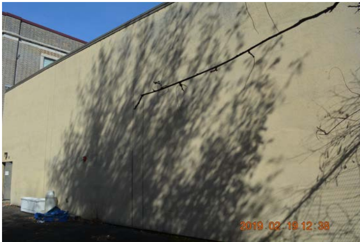
Photo 2: Pool facility exterior wall is constructed of concrete masonry units (CMU) in a bearing wall configuration, surfaced on the outside face with an Exterior Insulation and Finish System (EIFS).
