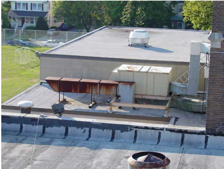
Photo 7: Eastern part of Pool Addition Roof: Roof over the pool space is the high portion beyond, in this view. The round roof top exhaust fan over the pool is visible. The lower section nearer and visible in this view is the area over the filter room before the white roof was put on in 2009.
